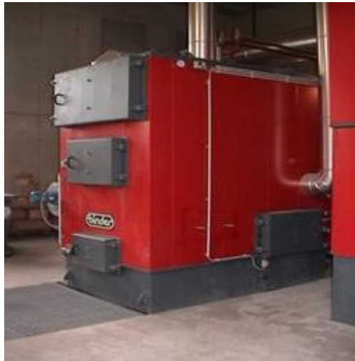
Photograph 3: Biomass Boiler
