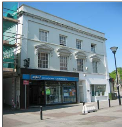
Before THI works
