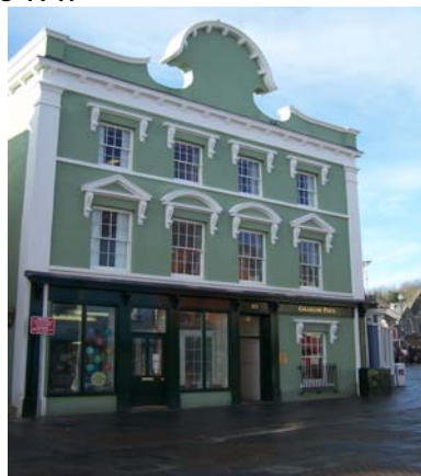
After THI works August 2007
