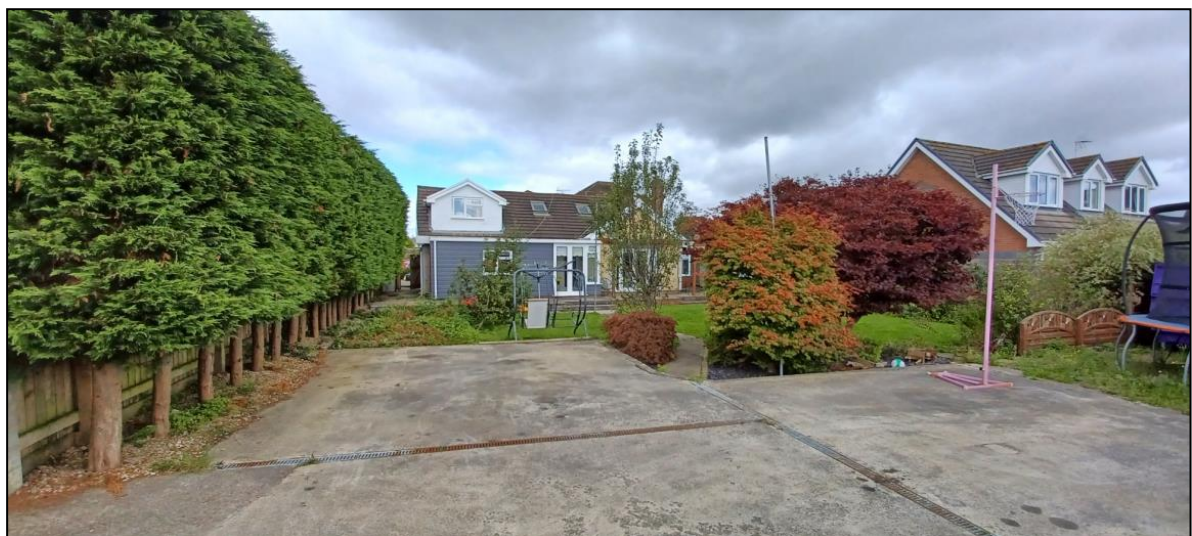
Figure 5 Rear Elevation of Application Dwelling
