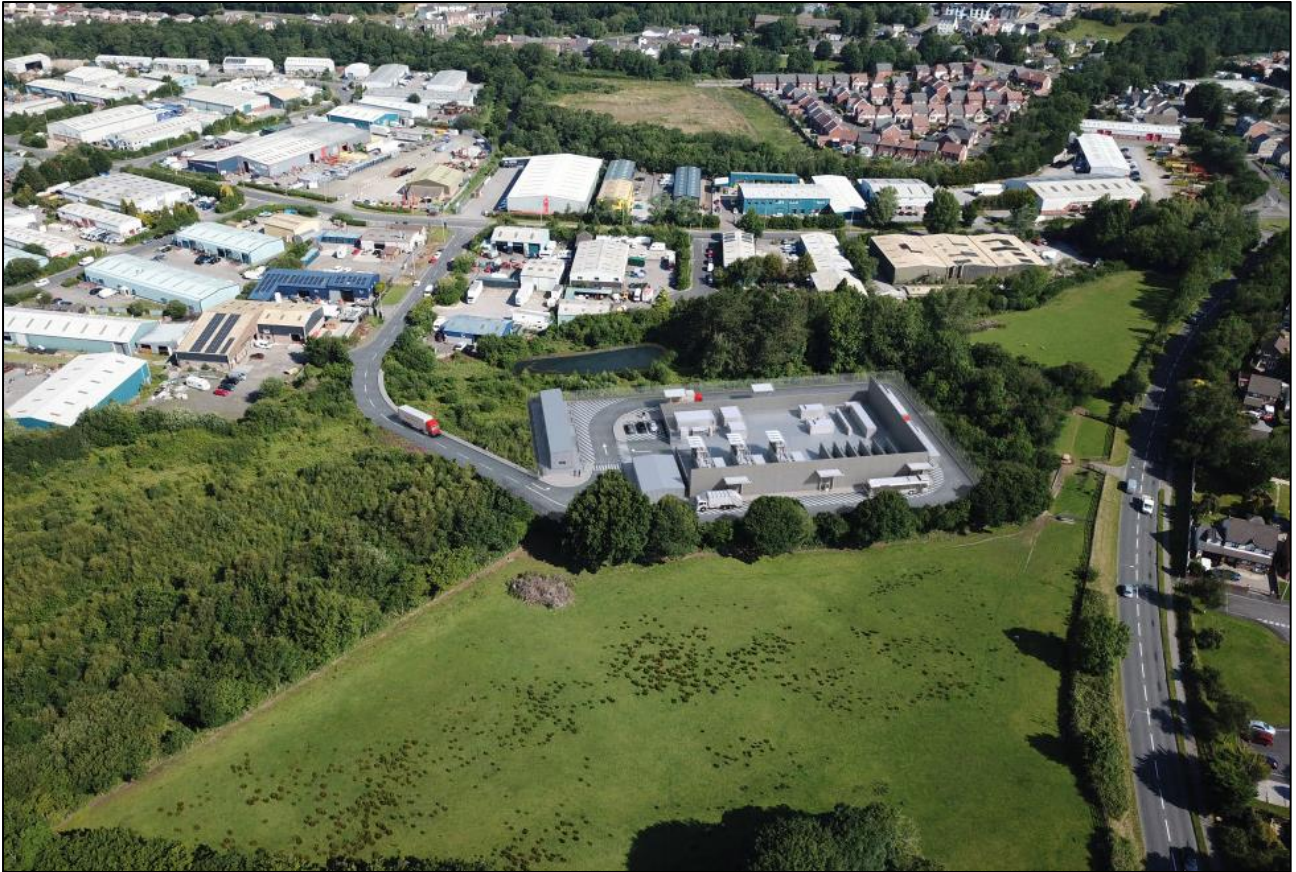
Figure 2: Birds Eye View of Hydrogen Production Facility inc.8 m High Wall and Immediate Surroundings
