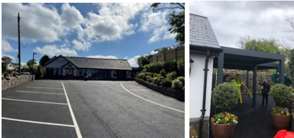
Figure 3 – Photographs of the application site
