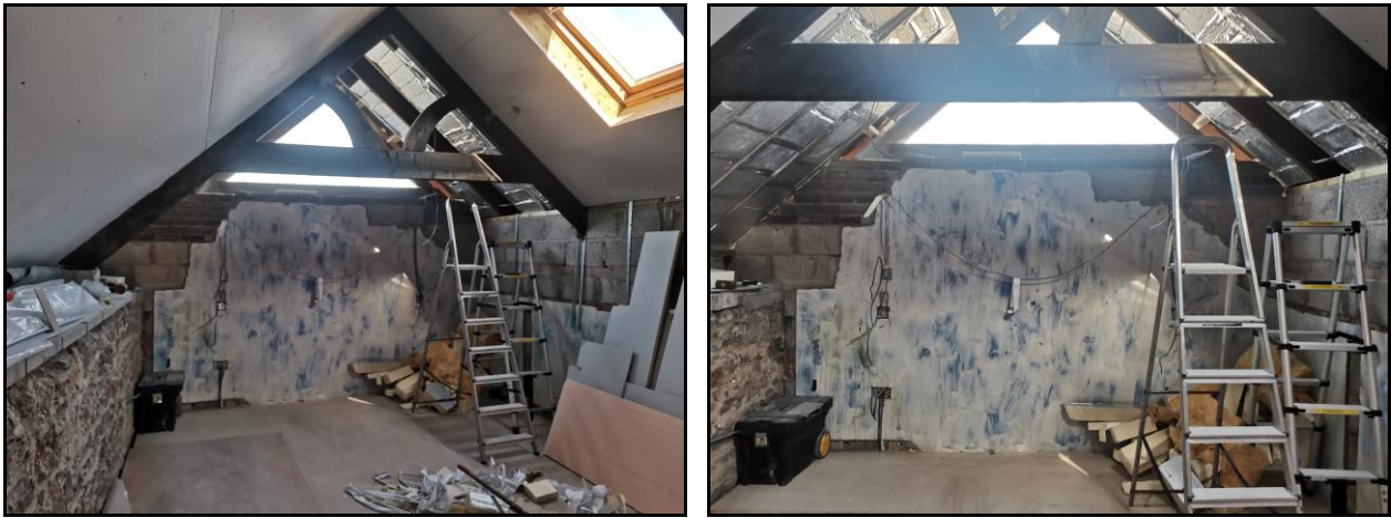
Internal Window Opening as built
