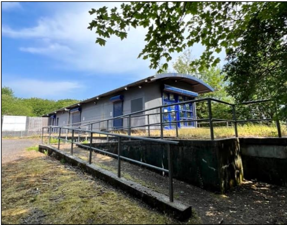
Figure 2 Photo of the Existing Office Building
