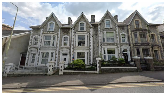
Fig. 2: Photo showing Front elevation of 61 Park Street
