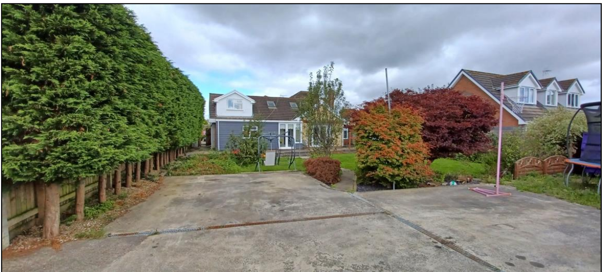
Figure 5 Rear Elevation of Application Dwelling
