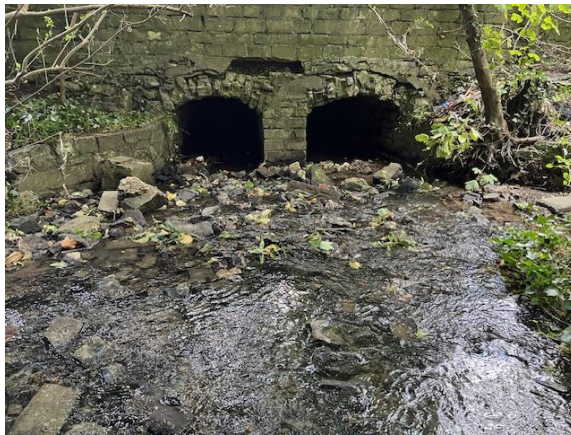
Figure 32 & 33 – Culverted watercourses Upstream of Oaklands Close
