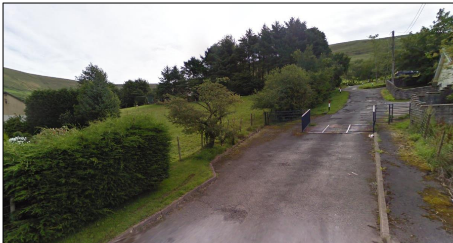
Figure 11: Photo of Site Frontage from 2010
