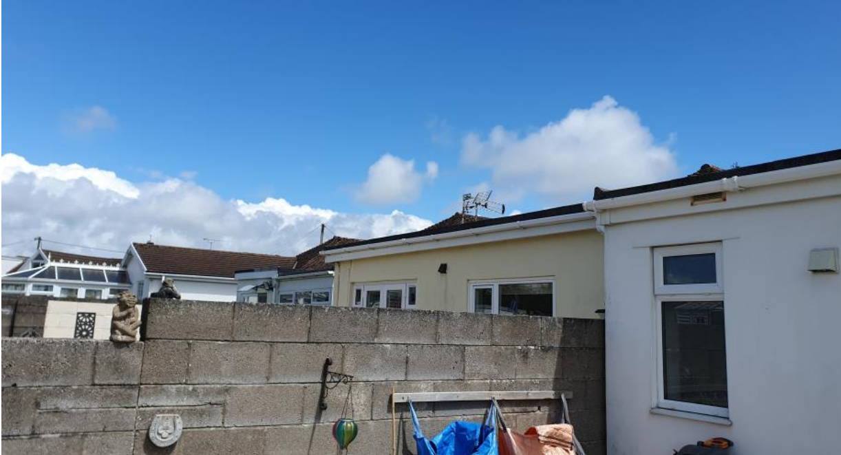
Figure 5 - Image showing other extensions
